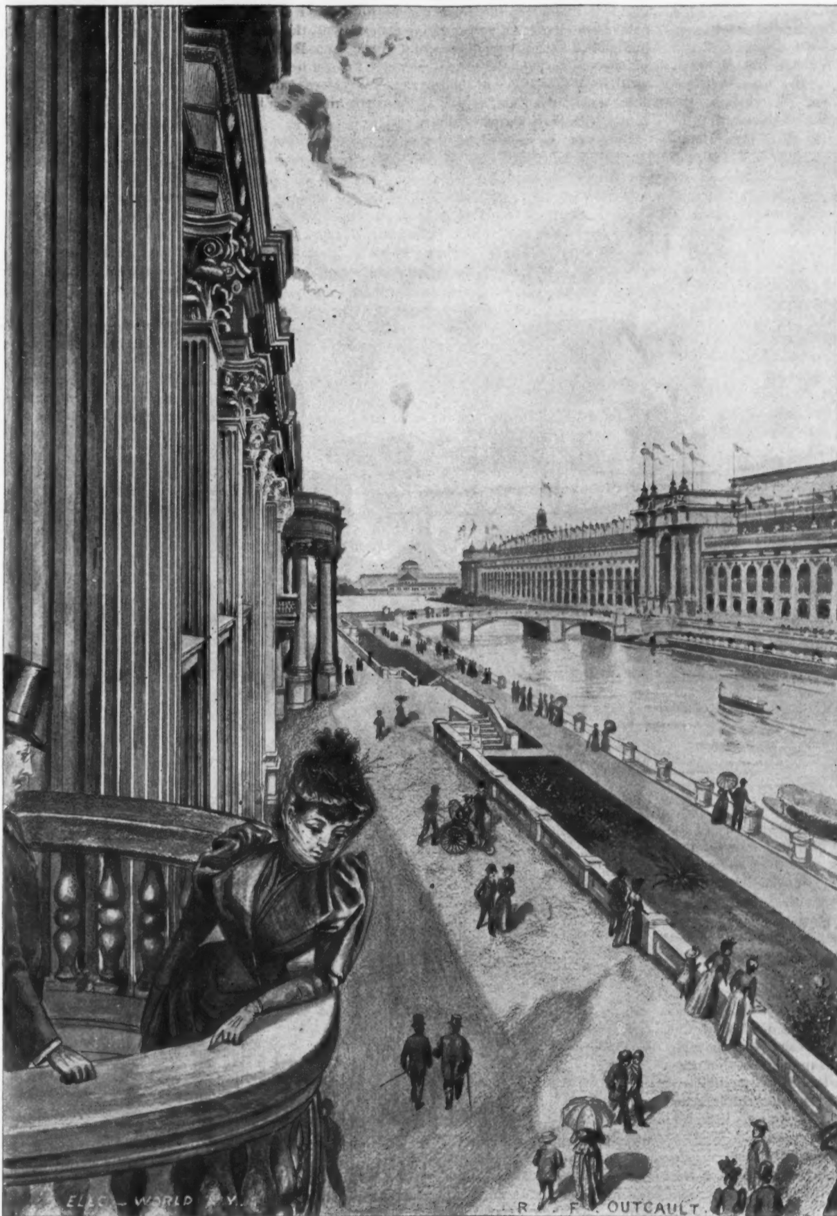
THE EAST FAÇADE OF ELECTRICITY BUILDING.
